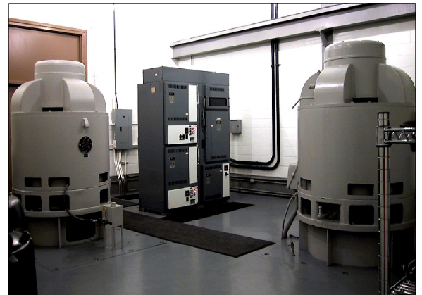
Spring Run pump station - Motor floor 2-350 hp motors with a pumping capacity of 47,500 gpm ea.
